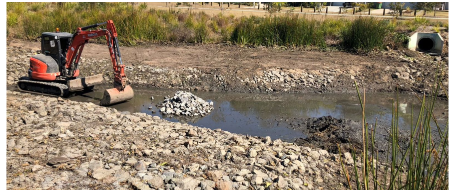
Yarrabilba sediment basin cleanout
